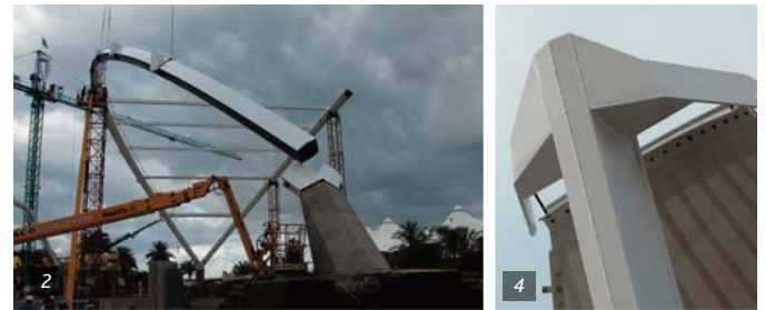
Figure 1. Steel structure. Figure 2. View during the installation of the arches. Figure 3. View during the assembly of the ribs. Figure 4. Masts used as fixing points for the semi conical membranes. Figure 5. Foundation wall and concrete piece. Figure 6. Roof view. Figure 7. Junction details.
